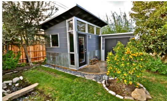
ADU in Los Angeles Photo courtesy of LADCP
