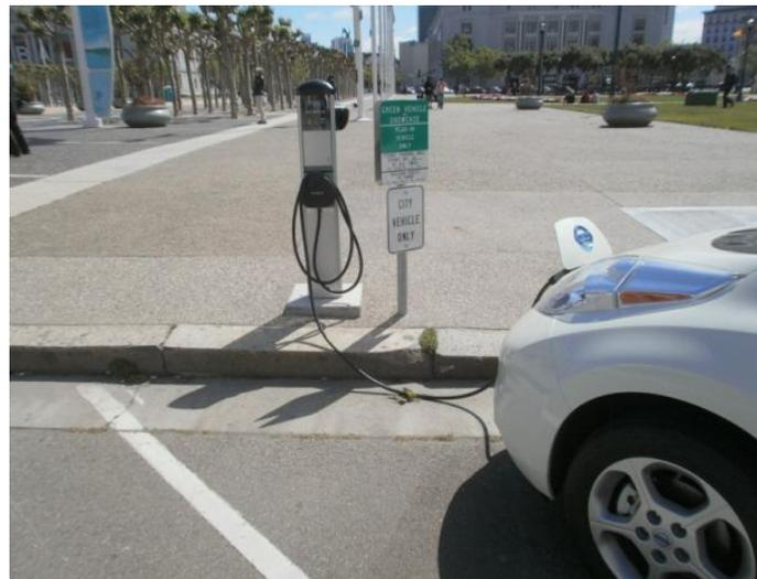
**Figure 24. On-Street E.V.C.S. (angle space, charger left of center)**
