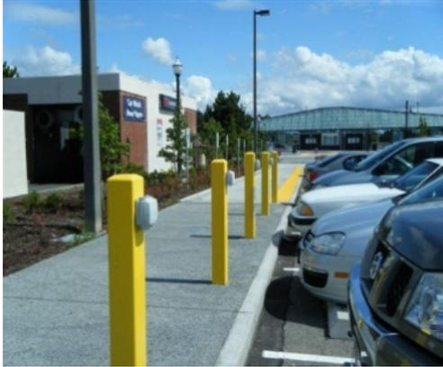
Figure 11. Series of 120V Level 1 Chargers in King County, Washington (entry sign-charging by reservation only)
