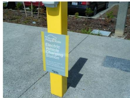
Figure 10. Non-standard E.V. charging sign on 120V Level 1 charging station in park-n-ride lot in King County, Washington
